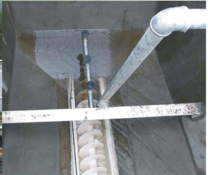
INCLINED GRIT COLLECTOR
