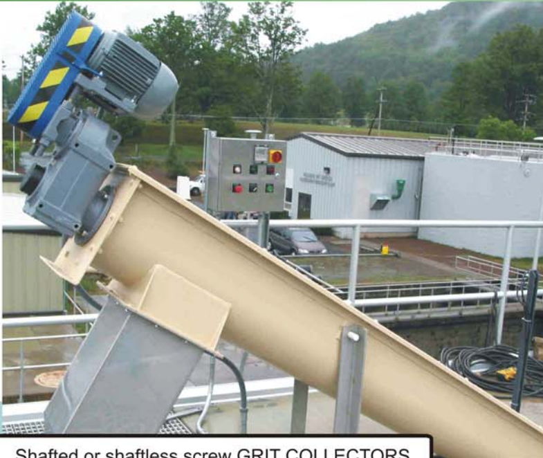
INCLINED GRIT COLLECTOR
